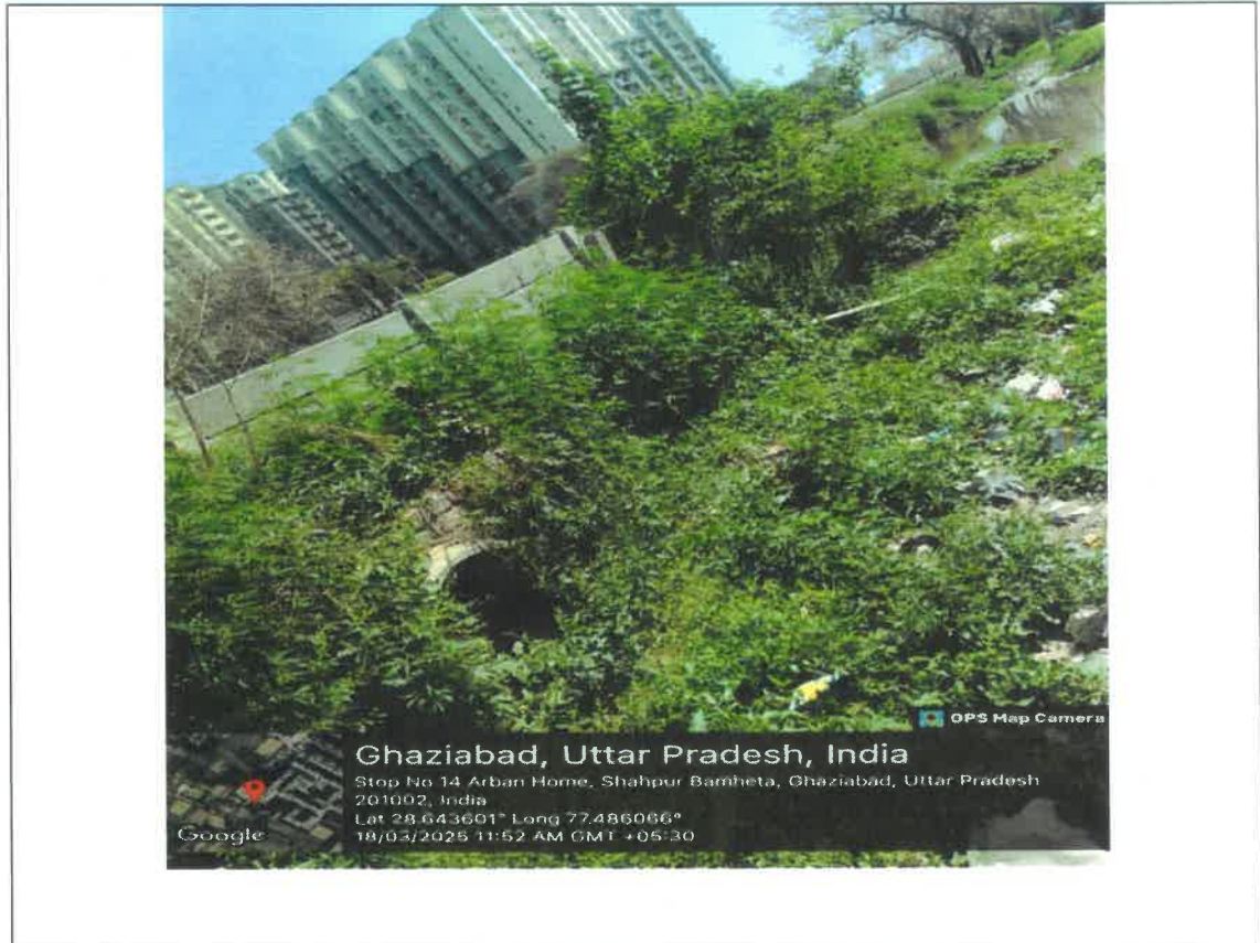
Pipeline near Group Housing Project Urban Homes
